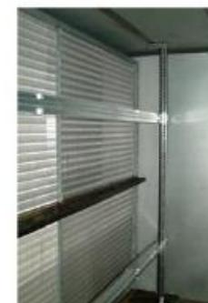
Fig. 8 Horizontal Lamp Placement for Coil Surface Disinfection
